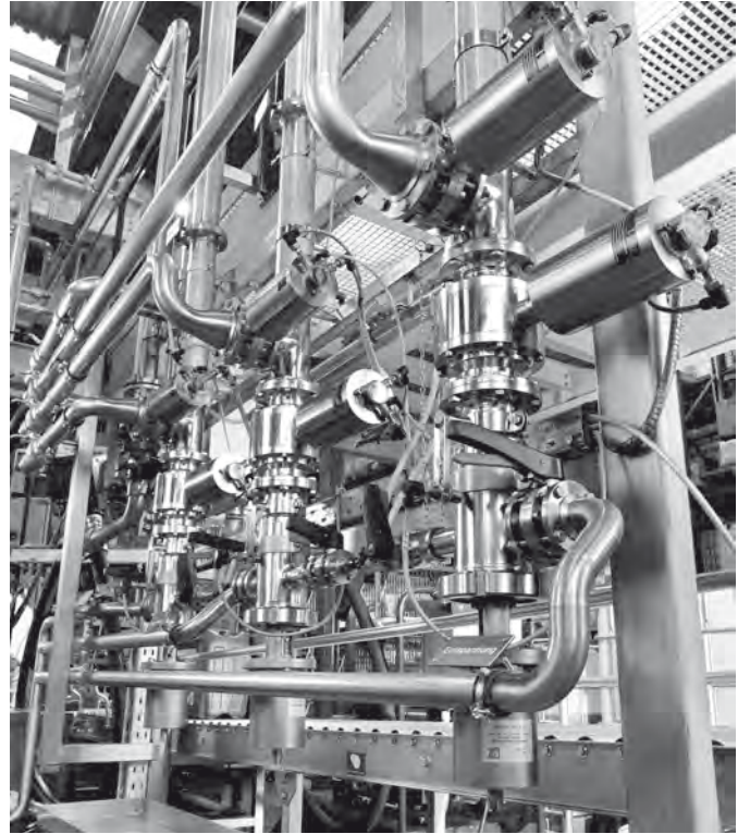
Guth Ventile pigging system in a production plant
